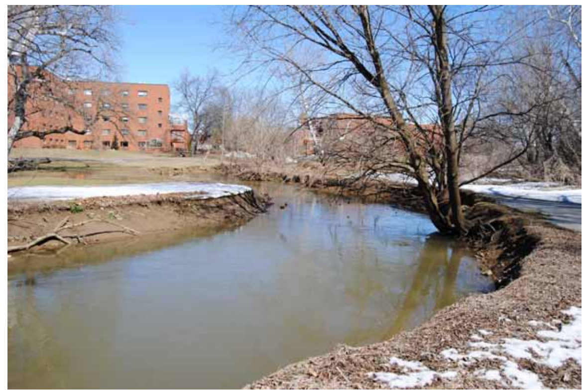
Existing stream channel and vertical banks
