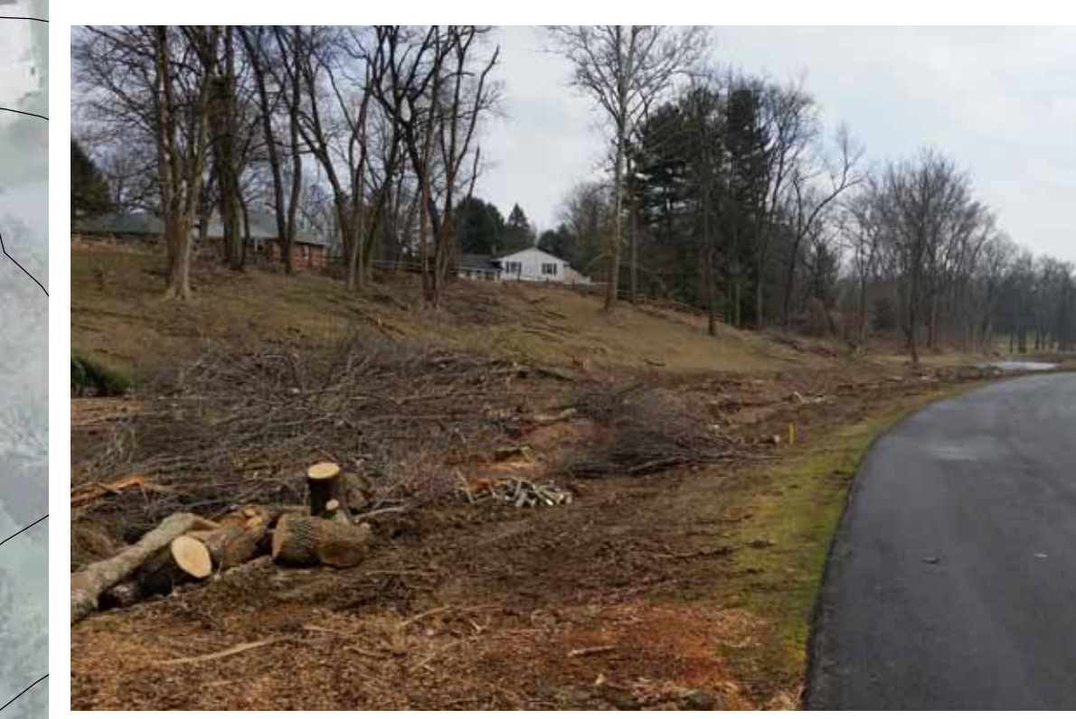
Eroded swale along entrance drive of Conestoga Country Club
